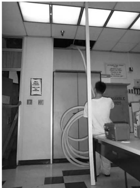
Figure 1. The cable pull. (Photo: Author)
